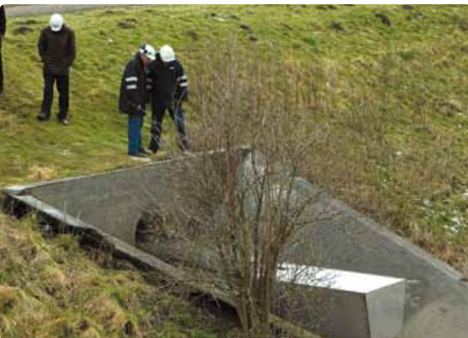
Filtering of waste water before discharging into water discharge area.
